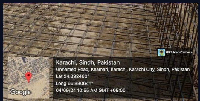
Site record, 4 September 2024 — reinforcement in place for the lined channel.
