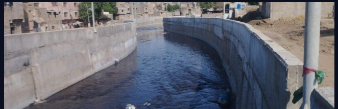
Existing condition — the lined channel and side road reserve along the Gujjar Nala corridor.
