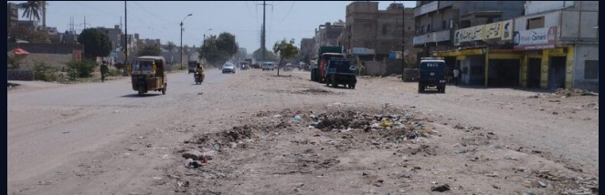
Existing condition — Road 13000, asphalt removed and subgrade exposed.
