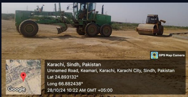
Site record, 28 October 2024 — grading and compaction of the subgrade at Keamari.
