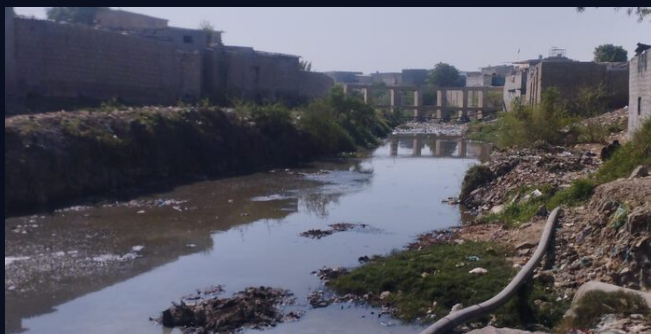
Existing condition — the unlined nallah where it runs through the built-up area.
